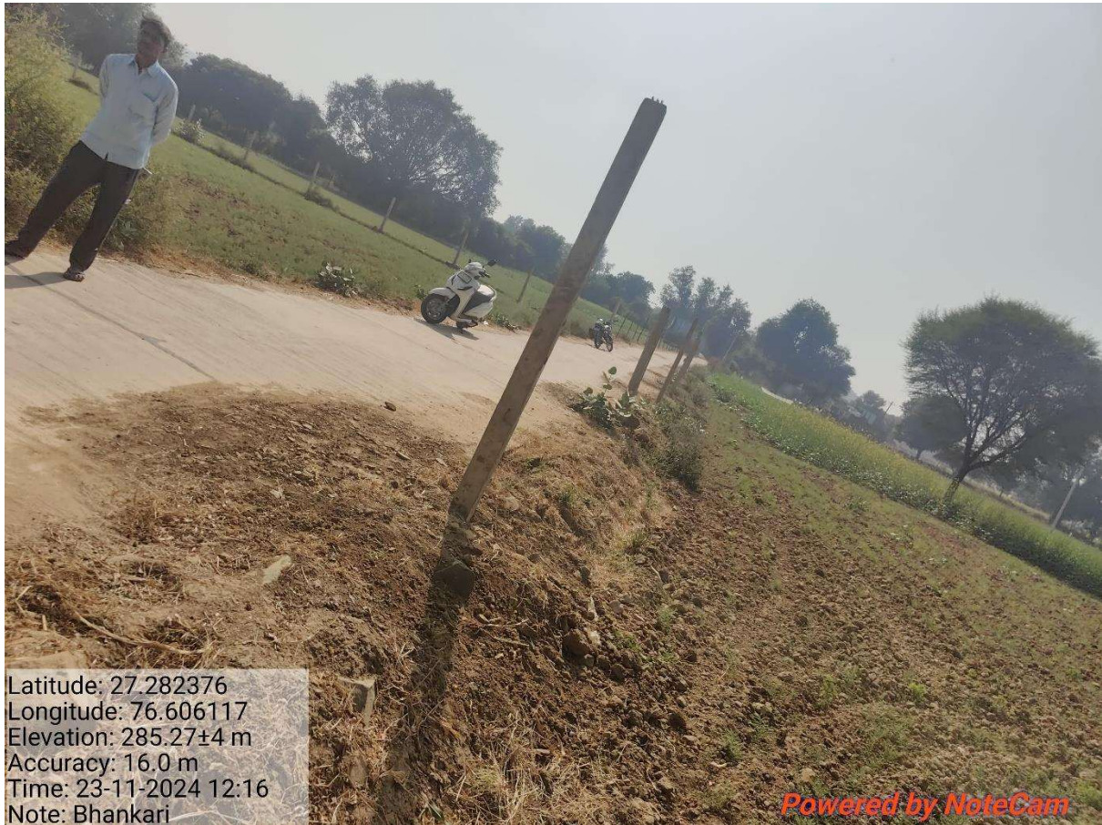
Figure 03: Newly constructed RCC road with no trees near applicant's fields where trees were uprooted
